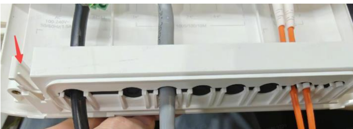
Figure3-11 Connecting Cables to the Equipment (8)
