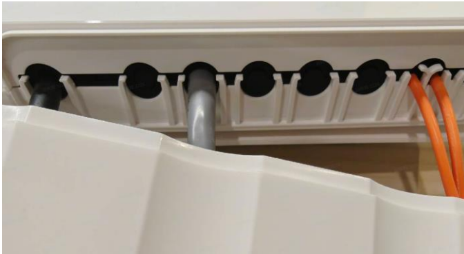
Figure3-12 Connecting Cables to the Equipment (8)
