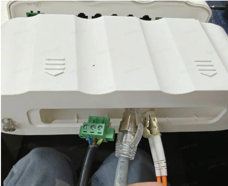
Figure3-7 Connecting Cables to the Equipment (4)
